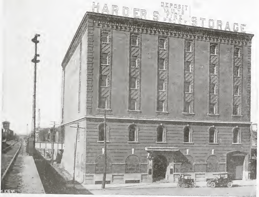
FIG. 4. HARDER'S FIREPROOF WAREHOUSE—CALUMET AVENUE BUILDING. Chicago, Ill.
